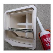
17. Seal the gap between the wall box and the telescoping adapter using a water prove sealant.
