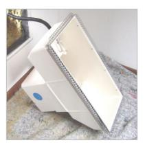
10. After the wall cut-out is completed install the electrical cable (3 x 1.5 mm<sup>2</sup>) in the upper part of the wall box. Affix the wall box flush with plaster and secure with wedges.
