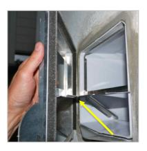
19. The metal outside air divider is attached to the telescoping adapter via 6 metal screws.
