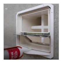
18. When installing the metal outside air divider make sure that the metal lip of the outside air divider seals properly against the interior air stream divider.
