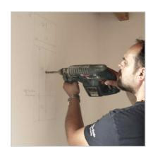
5. Sketch up the wall cut-out on the outside wall of  $27 \times 27 \text{ cm}$ .
