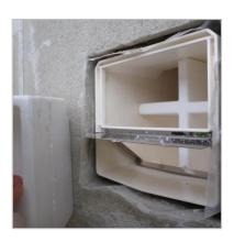
16. Install telescoping adapter flush with stucco. Use water prove sealant as shown.
